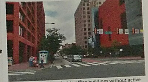
Independence Mall and wide office buildings without active ground floors make 2nd and 3rd Streets seem far away from Independence Hall and the East Market area about to undergo major reinvestment.
